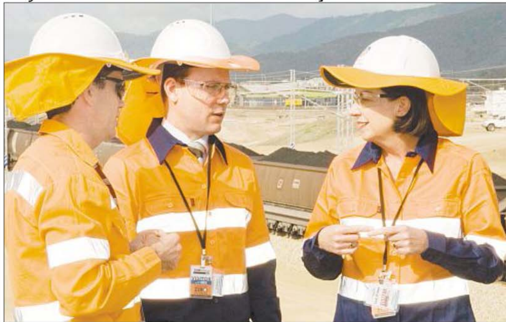
Inspecting the progress of the $500 million Jilalan Rail Yard upgrade south of Mackay are, from left, QR Network executive general manager Mike Carter, State Treasurer Andrew Fraser and Premier Anna Bligh.
